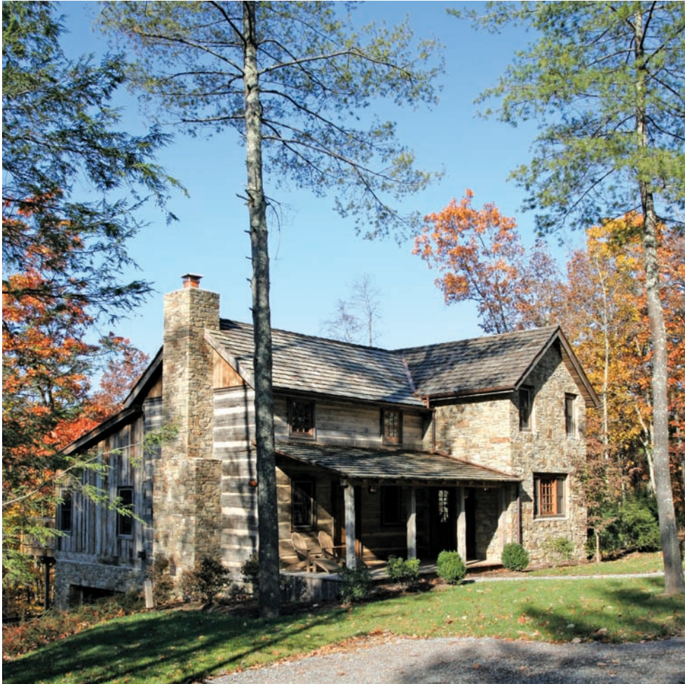
After nine years of looking, the Purdens fell in love with this cabin built from 150-year-old logs and now regard it as their own cozy getaway.
